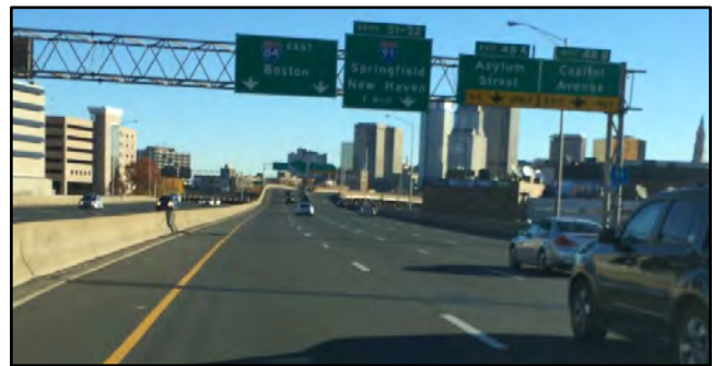
I-84 Eastbound – Two Basic Lanes & One Dedicated I-91 Lane with Two Lane Off-Ramp for Exit 48A&B
