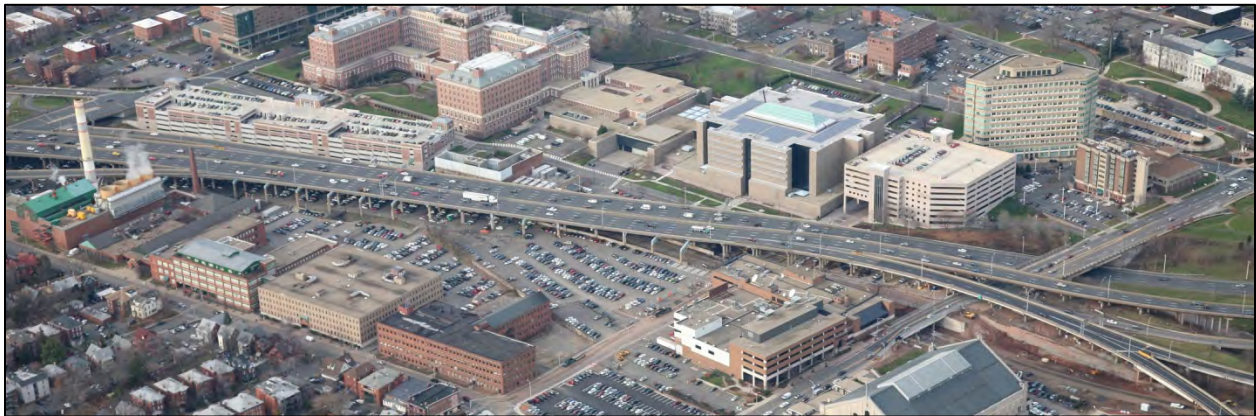
I-84 Viaduct Structures near Broad Street; Source: Skycomp, 2013
