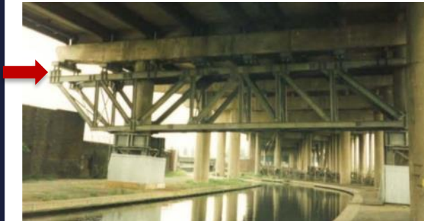
Temporary underpinning
