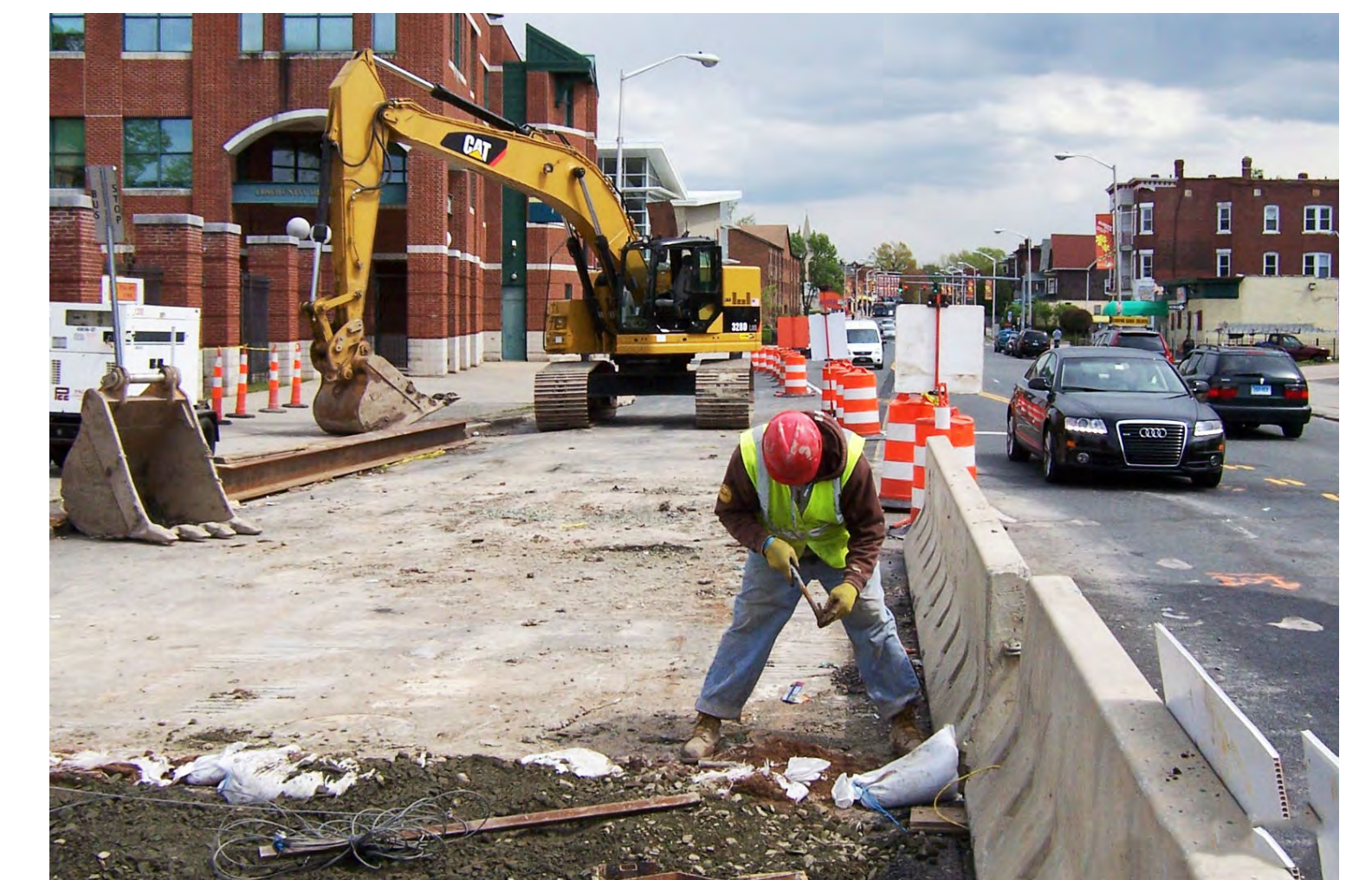
Conventional construction requires additional safety measures during construction
