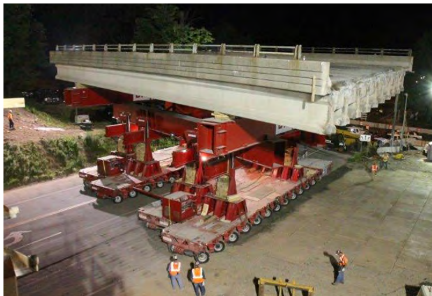
Example of Accelerated Construction Technologies on I-84 in Southington, CT
