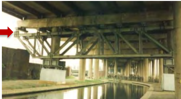
Temporary underpinning
