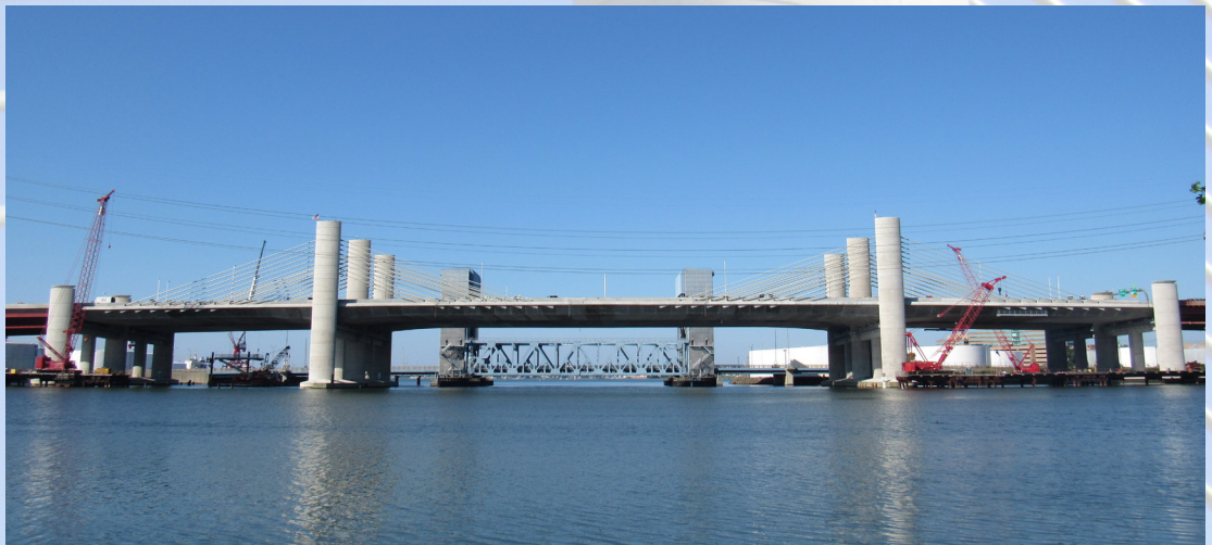
The Pearl Harbor Memorial Bridge, also known as the Q Bridge, crosses over Quinnipiac River between New Haven and East Haven. It is the nation's first extra-dosed bridge, combining cable stayed and box-girder designs for a striking and practical display of engineering.
