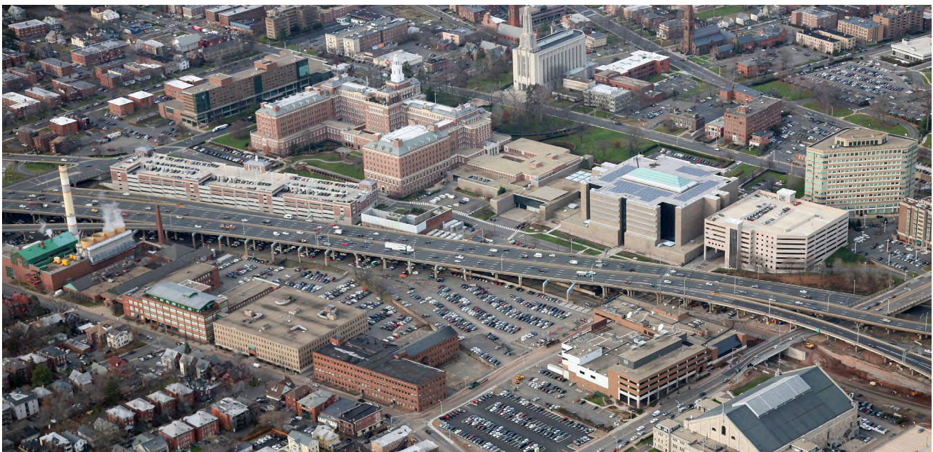
A portion of Hartford's I-84 viaduct from above.
