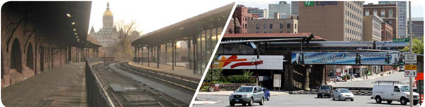
The rail viaduct, shown here from above and below, used to carry four tracks (two on each side of the Union Station platform). It now carries just one serviceable track.
