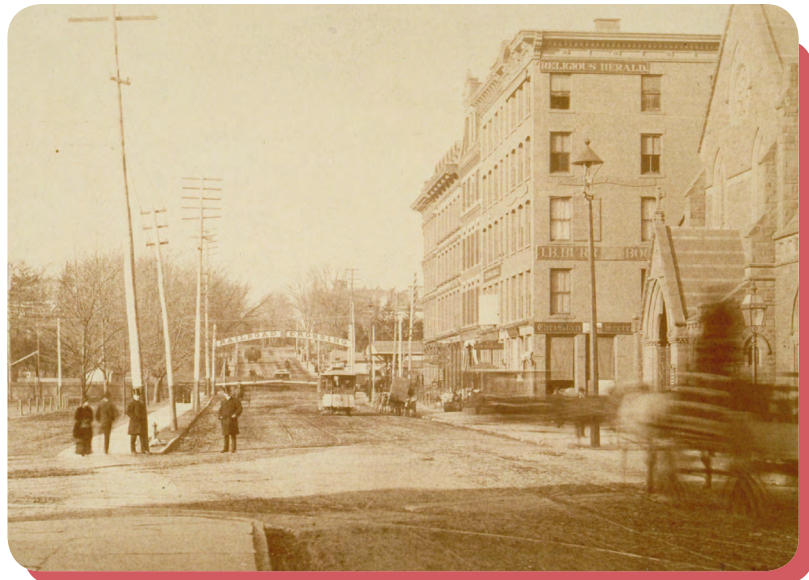
The railroad was originally constructed at-grade at Union Station, but the tracks were elevated in 1889 to avoid the heavy horse-drawn carriage traffic (and later, automobiles) on Asylum Street. The arch over the roadway is located where the rail viaduct now sits. (Photo courtesy of Archives and Special Collections, UCONN Library)
