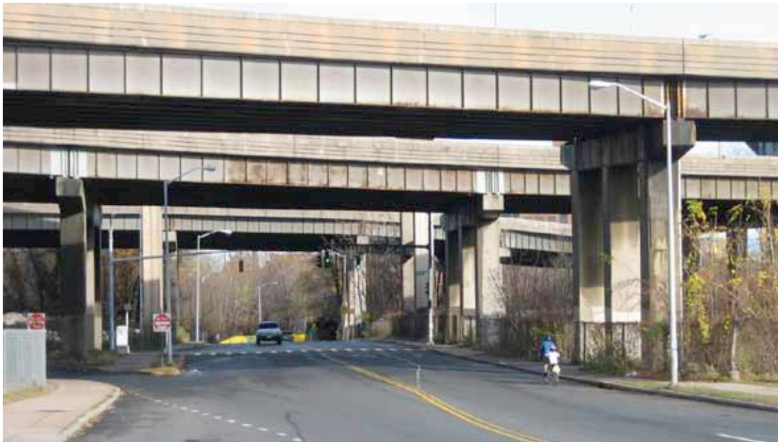
Capitol Avenue, near the Sisson Avenue interchange, passes below multiple highway ramps and the rail line, creating a sharply defined barrier between surrounding neighborhoods and downtown Hartford.
