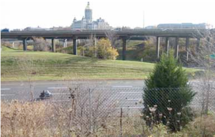
The Viaduct and its ramps divide the city—separating downtown and the Capitol from surrounding neighborhoods, and each other. Much valuable land is wasted.
